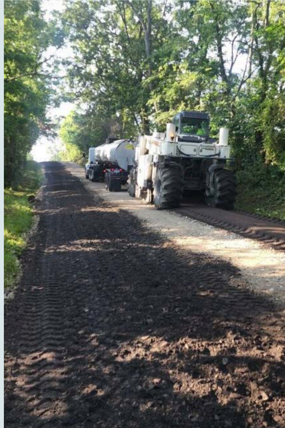
GRADING AND MIXING WITH OIL
