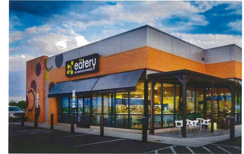
Reference Photo - Harmar Twp, PA
